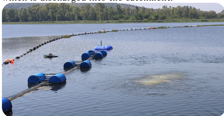
Part of the Hartbeespoort Dam, where the Nano Bubble technology is currently in implementation stage
