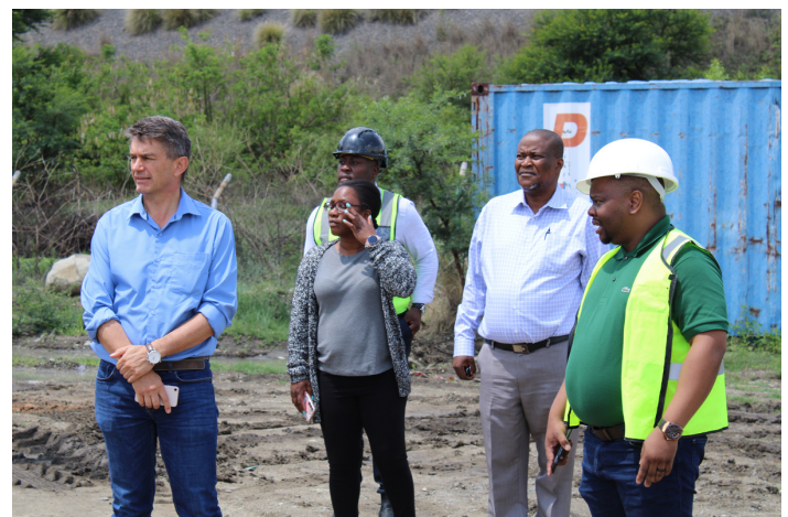
After the meeting, a walkabout was taken at the plant, to afford the appointed service an opportunity to assess the work done and take note of the challenges in respect of the unfinished work.
