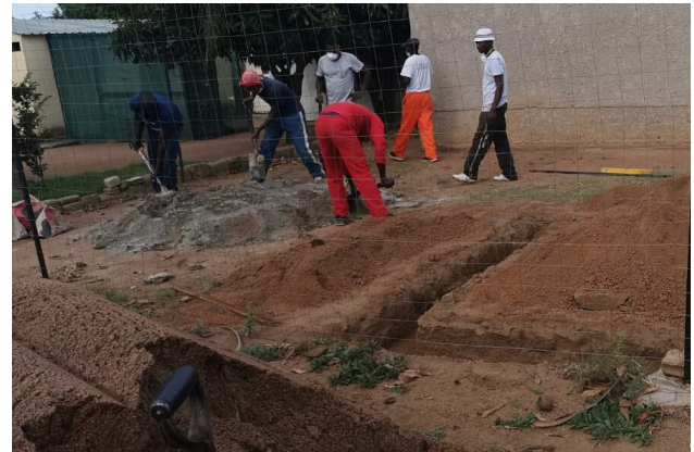
Magalies Water technical staff overseeing the construction of the stands in preparation for the installation of the water tanks in Lethlabile, Madibeng Local Municipality.
