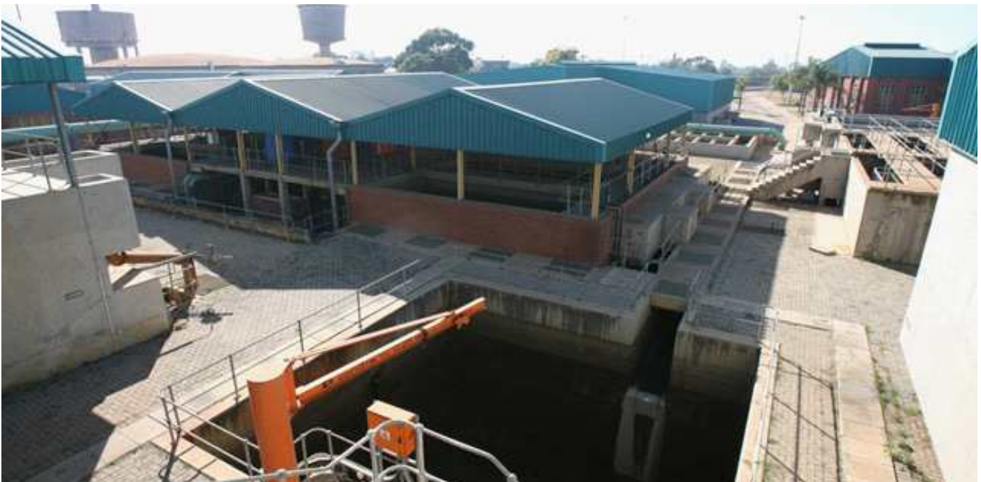
Figure 6: Temba WTP – 60ML/d Plant.
