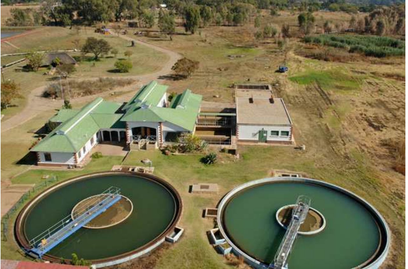
Figure 1: Cullinan WTP – 16ML/d Plant.
