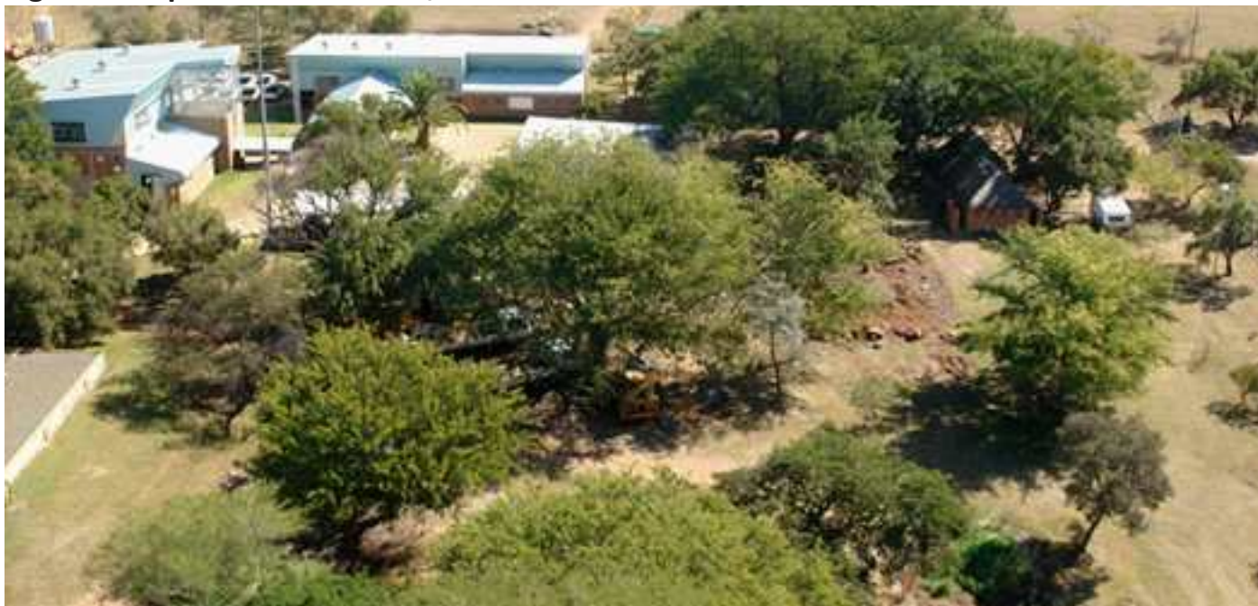
Figure 2: Klipdrift WTP – 18ML/d Plant.
