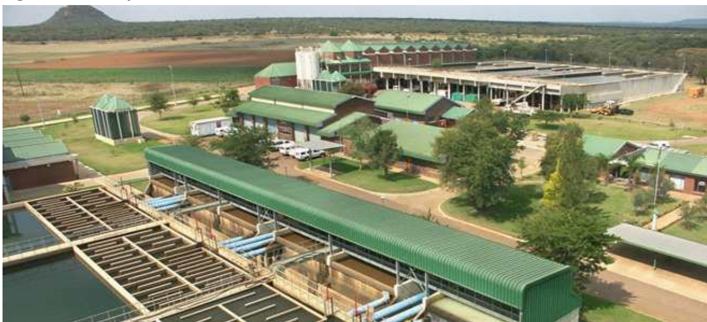
Figure 3: Vaalkop WTP – 210ML/d Plant
