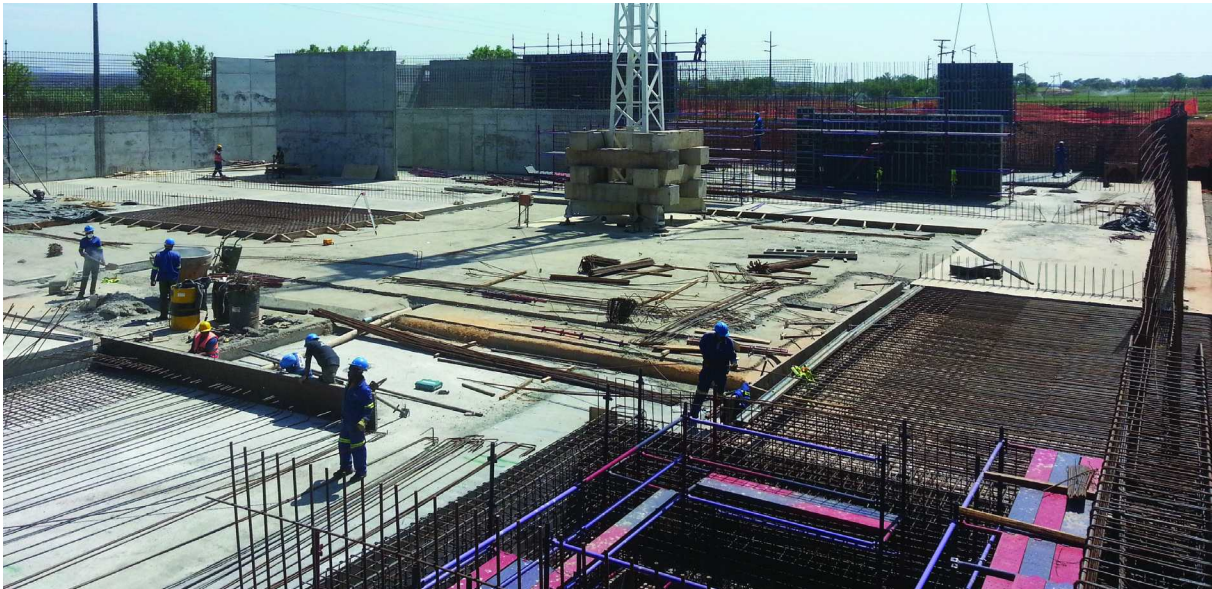
Construction of new filter beds at Vaalkop WTP
