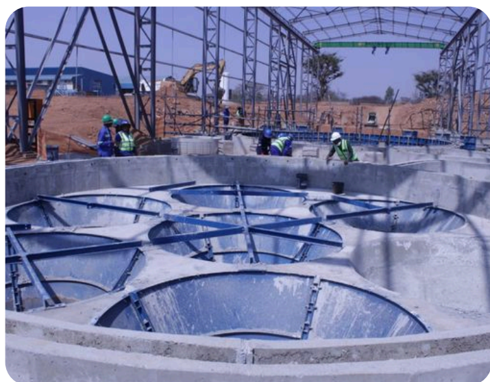
Longitudinal View: Construction Workers on site at the Klipdrift 50 Megalitre Package Plant
