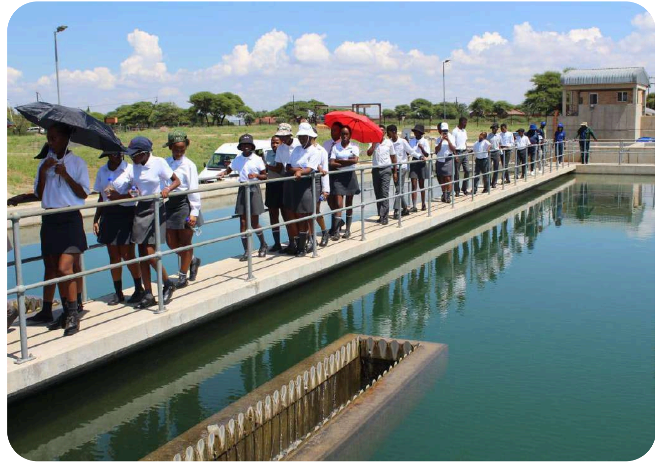
Maatla Secondary School learners taking a walk-about at the Taung Water Treatment Plant
